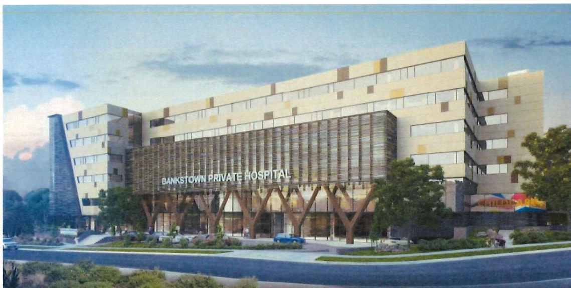
Figure 1: Bankstown Private Hospital concept viewed from Mavis Street (FSR of 2.73:1 is shown).
