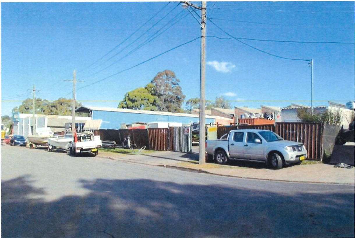
Figure 5: View of the site from Mavis Street.
